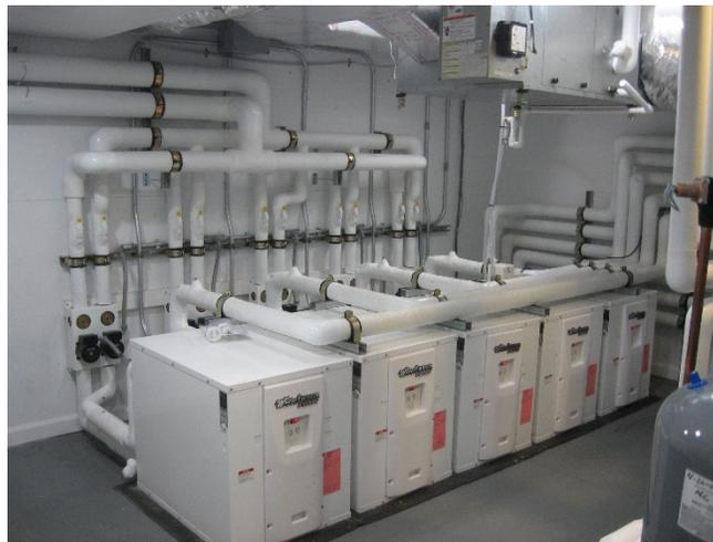
Condensers and other air conditioning equipment are usually mounted outside on the roof of buildings. GSHP systems do not require this and as such, structural and architectural building cost savings are realized.
